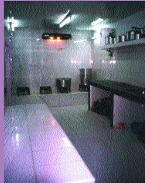
KITCHEN AFTER RENOVATION, HOTEL MOUNIA, FES, MOROCCO
