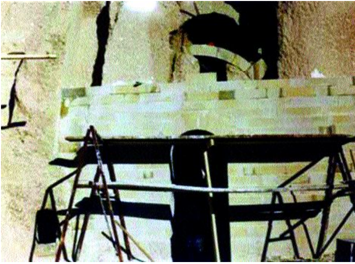
EXTERIOR VIEW OF THE SARICA CHURCH DURING RESTORATION
